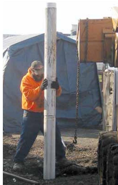
A worker closing a well that removed diesel fuel from the groundwater.
